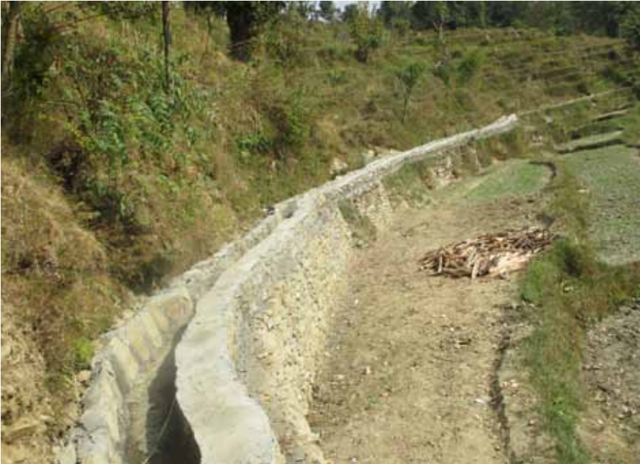
Newly rehabilitated irrigation canel
