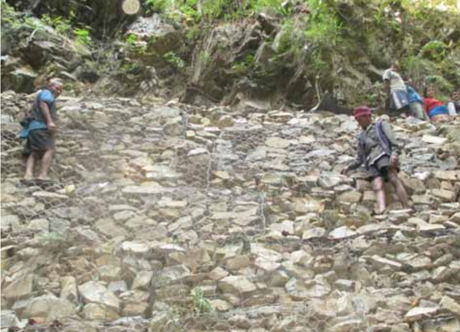
During Construction of gabion walls
