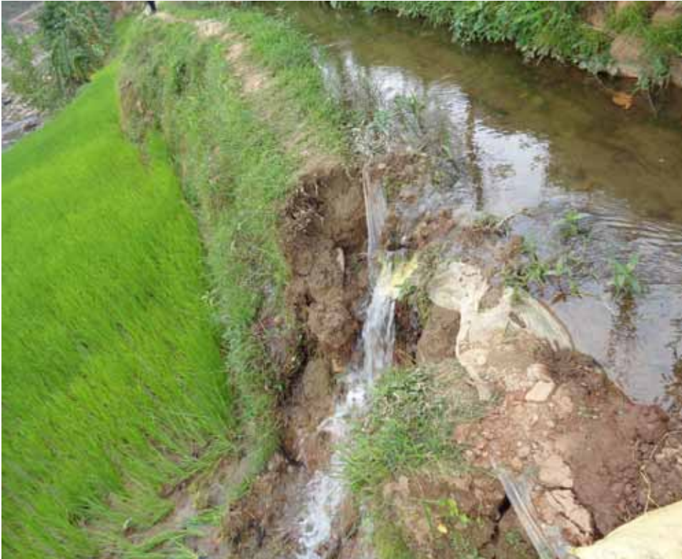
Damaged irrigation canal after the earthquake
